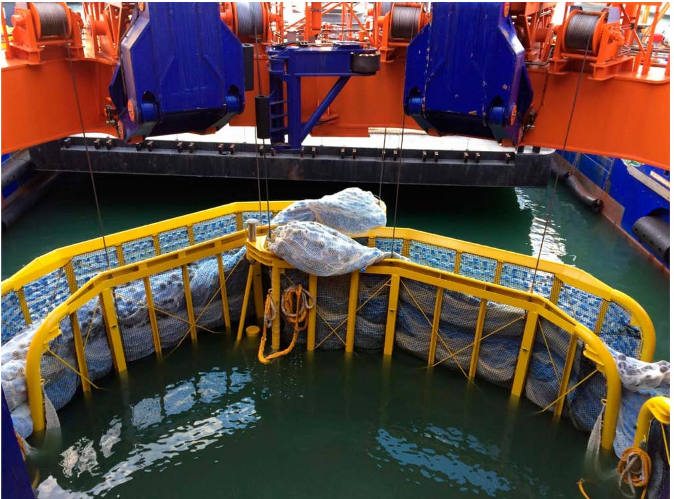
**FIGURE 6.** EXAMPLE OF A NOISE-ABSORBING HSD (HYDRO SOUND DAMPER) DEVICE PLACED AROUND A SEABED PILE FOUNDATION DURING INSTALLATION (SOURCE: VAN OORD).
