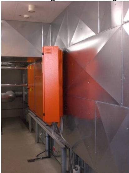
**Figure 3-27: Exhaust air heat exchangers at Ridelberg school**
