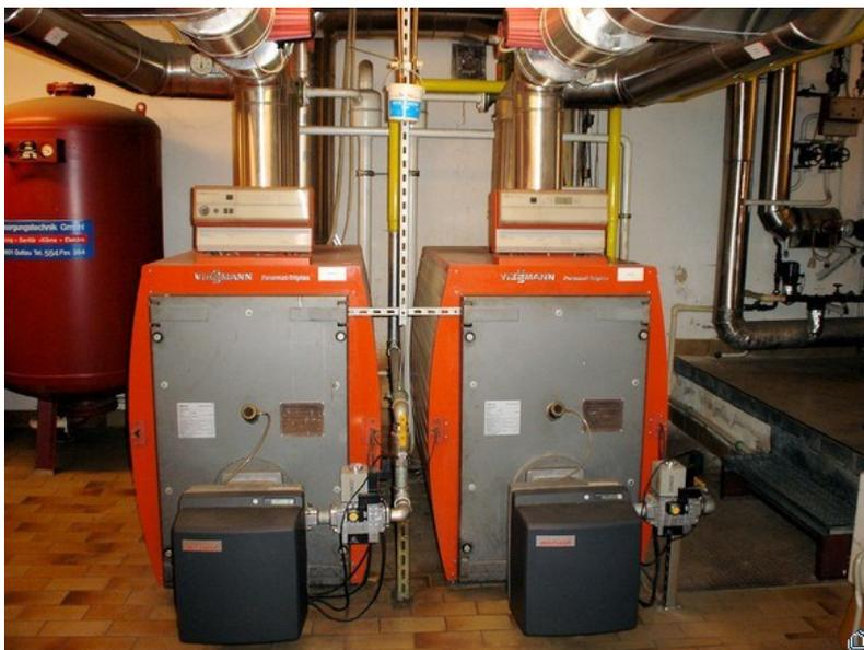
**Figure 3-21: Gas boiler providing heating before renovation of Olbersdorf school (EnOB, 2010)**
