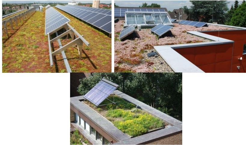
**Figure 6-9: Combination of green roofs and PV panels; on the right picture a solar thermal panel is presented**
