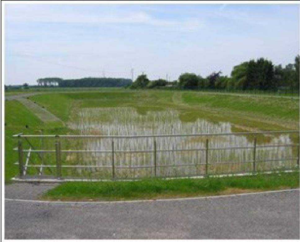
**Figure 11-31: Retention basin (sedimentation) and retention soil filter for the disposal/treatment of storm water**
